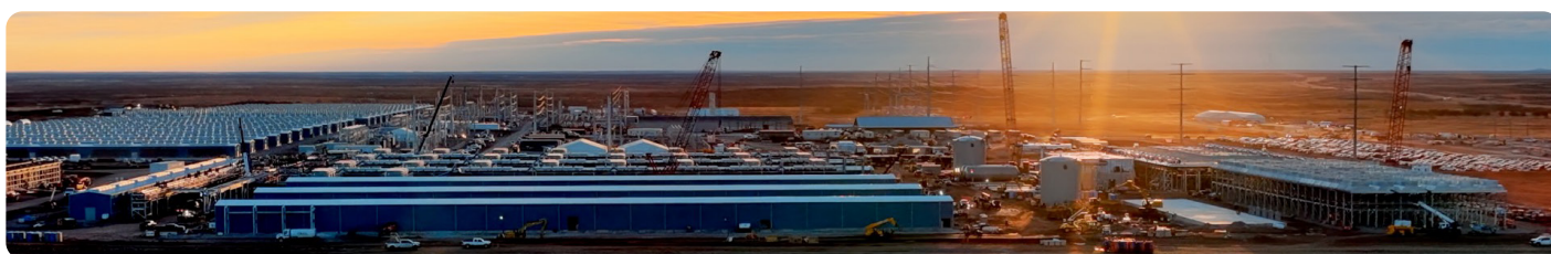
IREN Data Centre in Childress, Texas.
